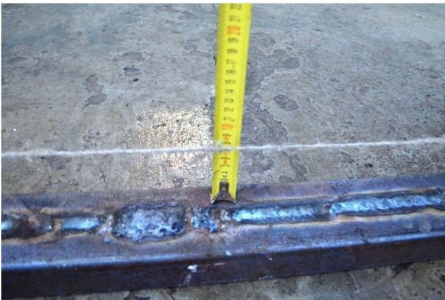
Fig. 3.8. Measurement of deflection in mid-span
