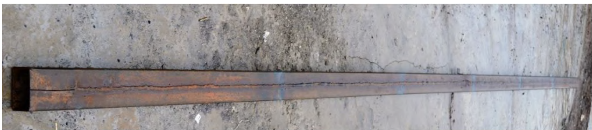
Fig. 3.14. Beam after thermal straightening
