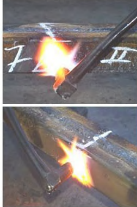
Fig. 3.12. Heating of wedges with gas burner
