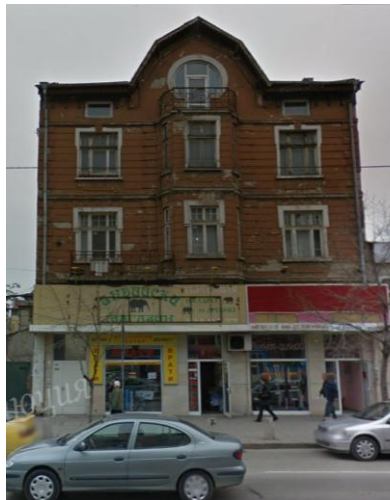
2 Frontal entrance facade Picture from 2012
