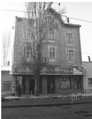
1 Frontal entrance facade Archive picture from NAG- Sofia
