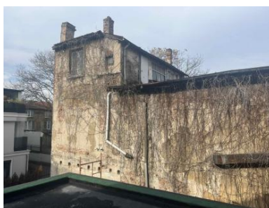
4 Side -facade-2025 (no traces from pre-existin windows)
