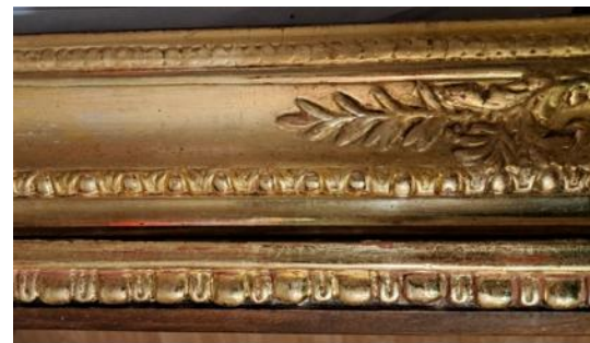
Figure 19. Tinting of matte gilding scuff areas on matte gilding loss areas and glossy gilding restoration on the door frame egg-end-darts
