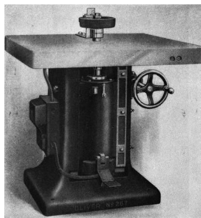
7. *Boring machine* was designed to hold and operate various wood bits. The single spindle manually operated borer is most adaptable for the general wood shop. It consists essentially of a frame or column, boring head, table, and various machine wood bits.
