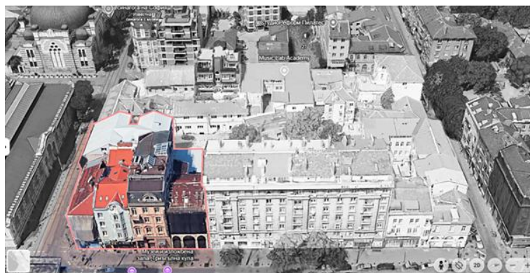
Figure 3. Building authenticity in bigger scale- the Spatial Void
