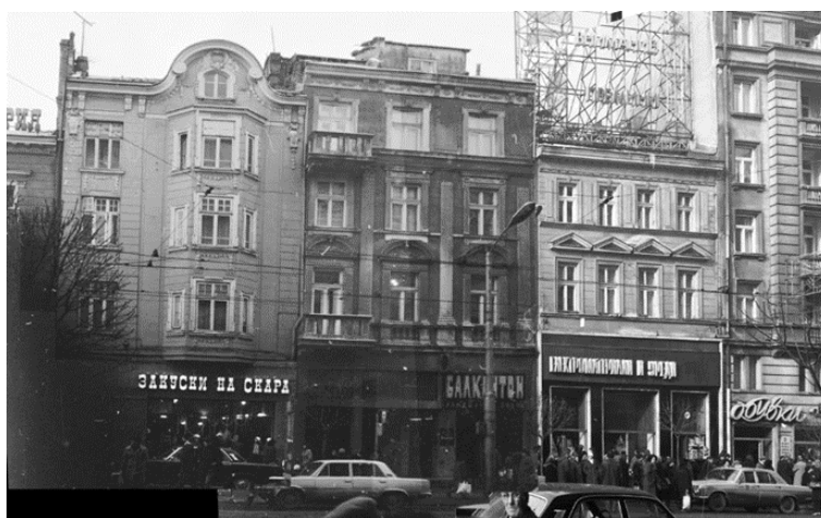
Figure 2–5. Stages of construction and silhouette interventions. 1970–80.
