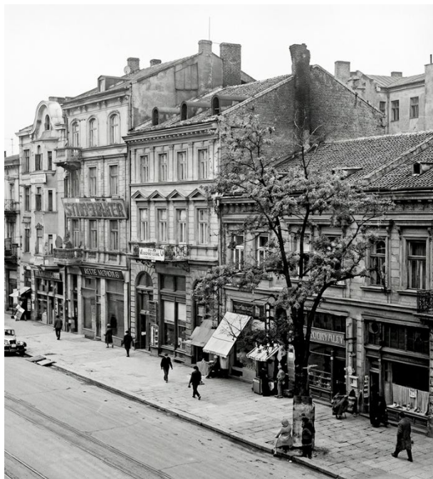
Figure 2–4. Stages of construction and silhouette interventions. 1940. Restored.
