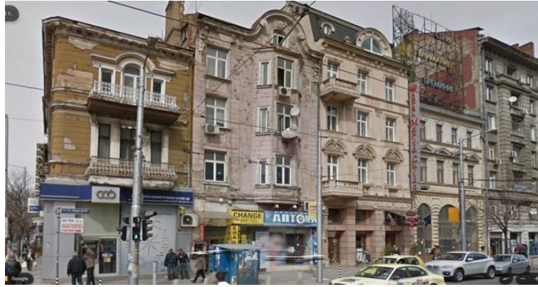
Figure 2–6. Stages of construction and silhouhette interventions. 2012.
